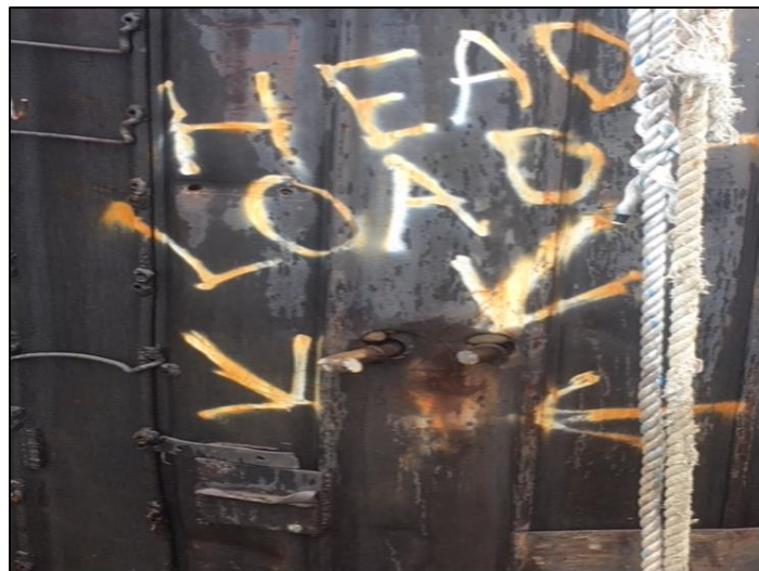
At left, a piling with mooring rings as designed. At right, the forward piling with a broken mooring ring anchor point and missing ring.
