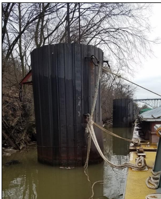
Mooring cell at the Jacks Run fleeting area. (Photo by Coast Guard)
